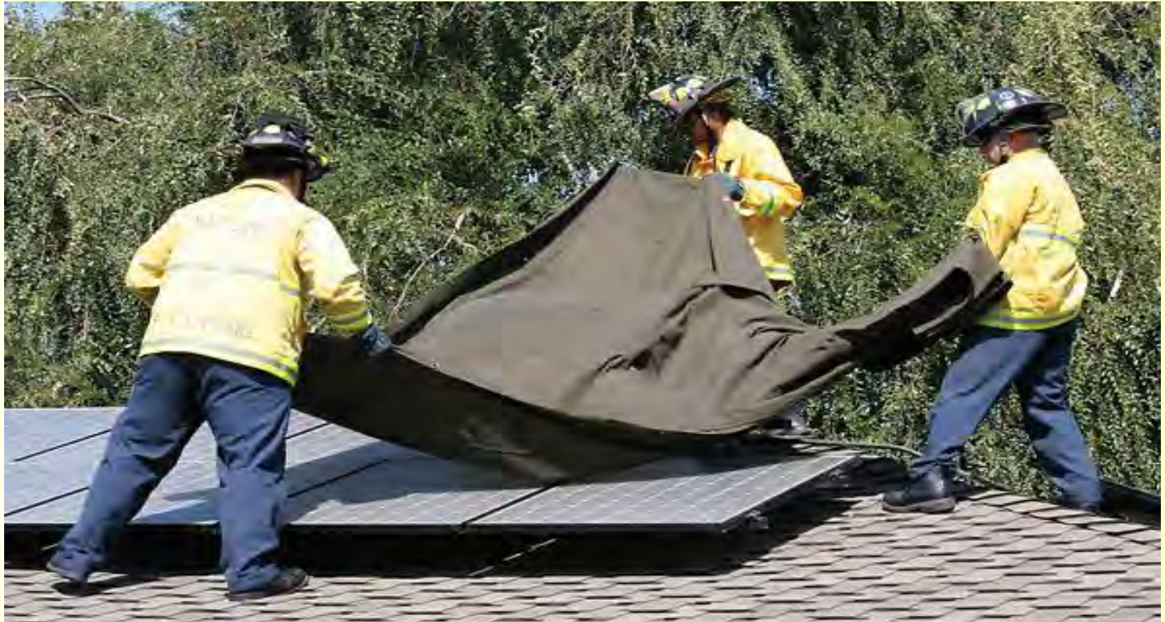
Covering panels with a heavy tarp is one approach that firefighters use to reduce voltage on a PV system (Photo courtesy of Matthew Paiss, San Jose (CA) Fire Department).
