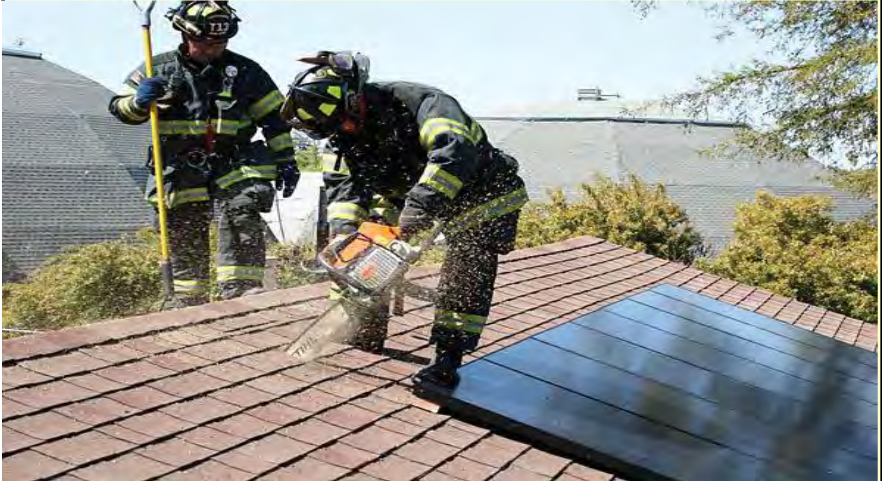
Firefighters typically use rooftop venting techniques when battling a blaze (Photo courtesy of Matthew Paiss, San Jose (CA) Fire Department).
