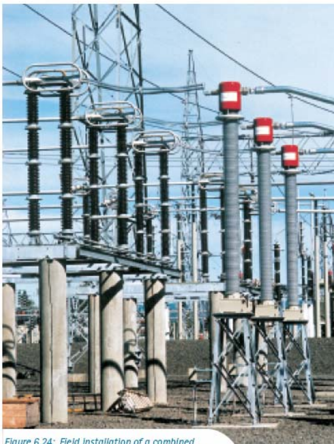
Figure 6.24: Field installation of a combined optical CT/VT
