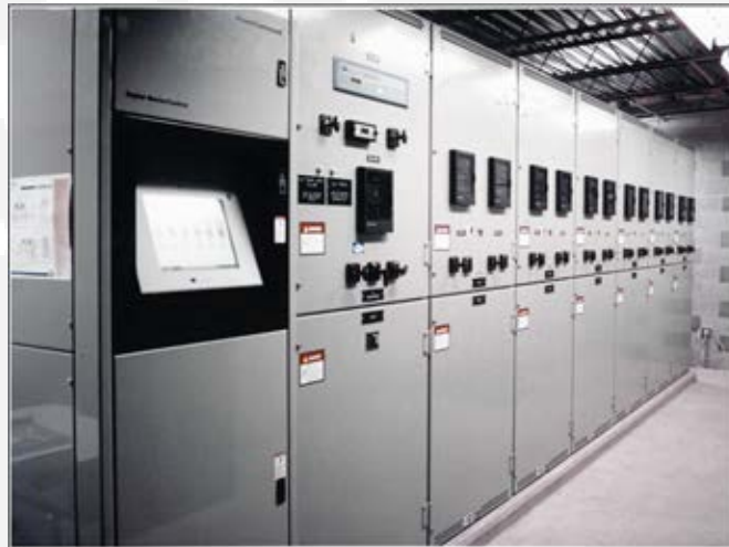
FIGURE 47. MEDIUM VOLTAGE PARALLELING SYSTEM WITH MASTER CONTROL.
