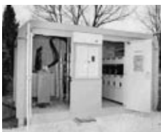
Fig. B38 : The four designs according to IEC 62271-202 standard and two pictures [a] walk-in type MV/LV substation; [b] half buried type MV/LV substation
