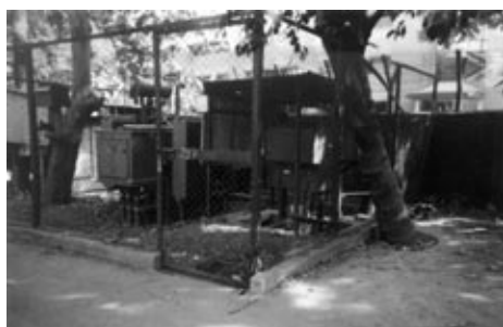
Fig. B39 : Outdoor substations without enclosures
