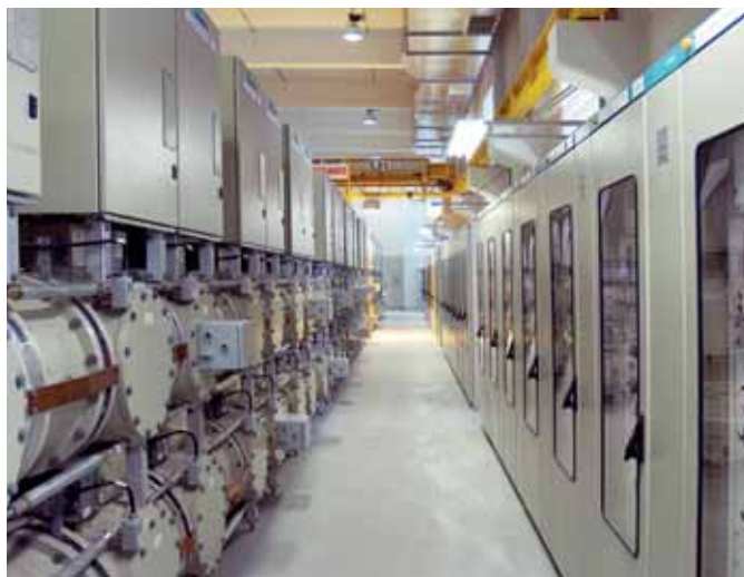
Fig. 3.1-34: 8DN8 GIS for a rated voltage of 145 kV
