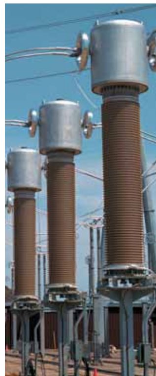
Fig. 4.5-3: 550 kV gas-insulated current transformer
