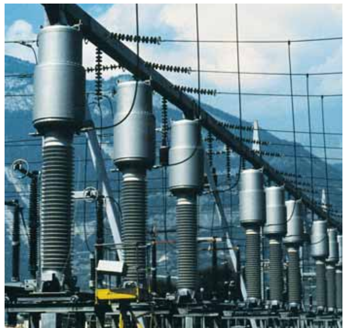
Fig. 4.5-9: 245 kV gas-insulated combined instrument transformer
