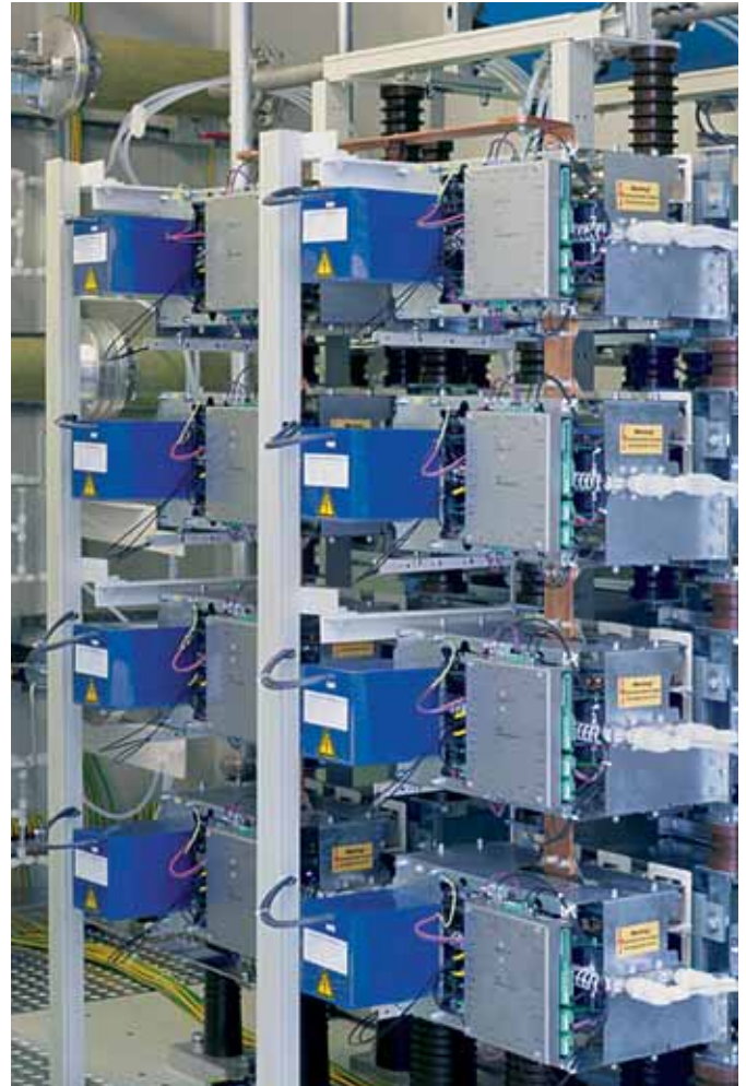
Fig. 2.4-3: IGBT converter of the SVC PLUS
