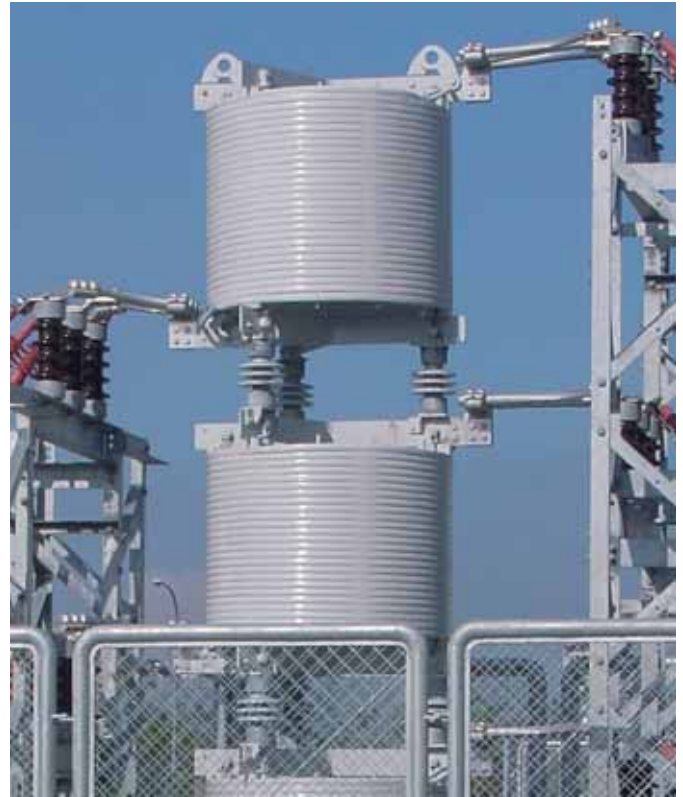
Fig. 4.6-2: 3-phase stacked current-limiting reactor
