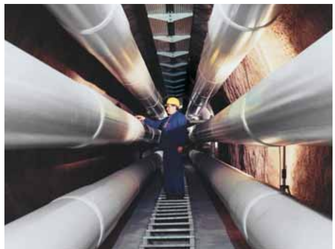
Fig. 2.5-1: GIL arrangement in the tunnel of the pumped storage station in Wehr, Southern Germany (4,000 m length; in service since 1975)
