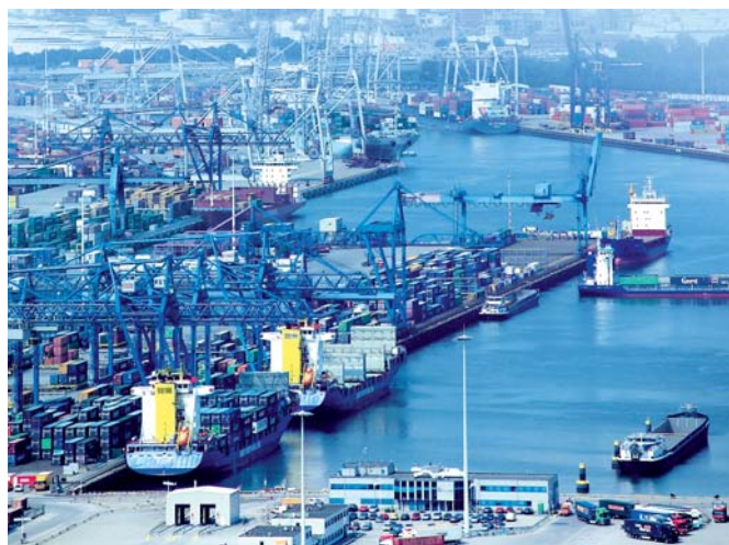
Fig. 2.3-3: An innovative solution to counter “harbor smog”: Siemens technology supplies ships in port with environmentally friendly electricity from the public network
