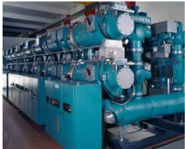
Fig. 3.1-37: 8DN9 switchgear for a rated voltage of 245 kV
