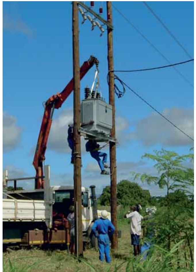
Fig. 5.9-1: Pole mounted, USA
