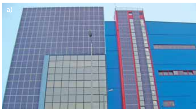
Fig. 2.7-1: Example of photovoltaic system: a) Facade-integrated PV system in Italy b) Installation of an earth-based PV system of 1 MWp in Italy c) Example of a 30 m high stadium roof system
