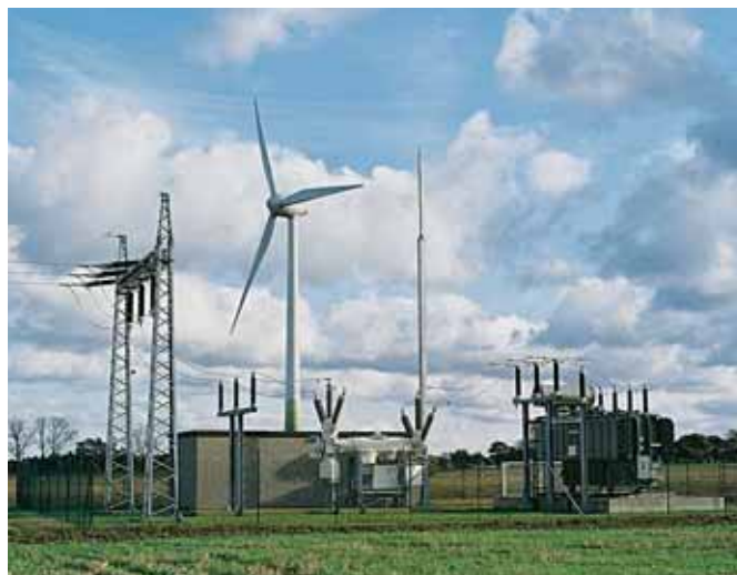
Fig. 3.1-35: 8DN8 HIS for a rated voltage of 145 kV
