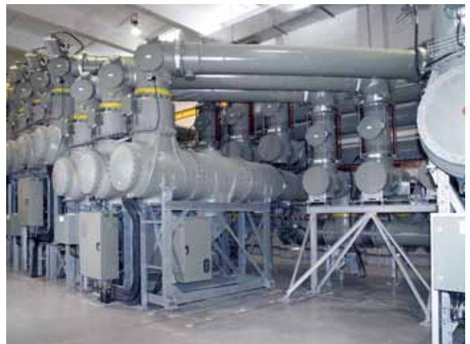
Fig. 3.1-49: The 8DQ1 modular system can meet customer requirements with just a few components.
