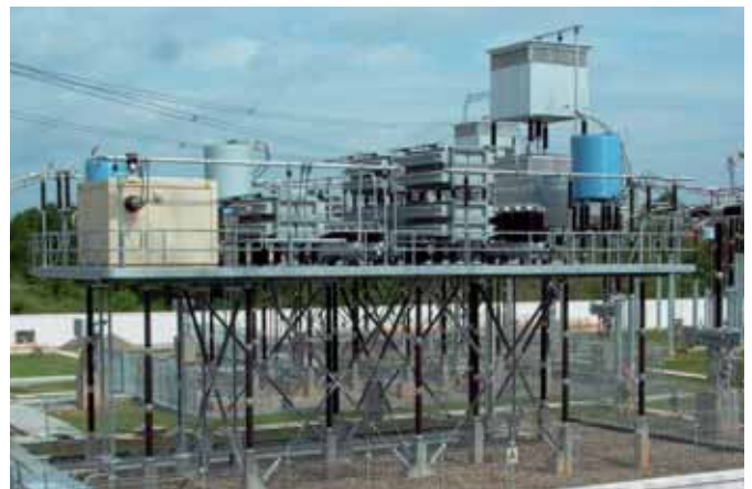
Fig. 2.4-5: View of a TCSC system
