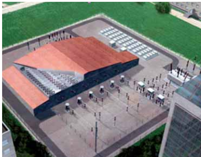
Fig. 2.2-8: Design of an HVDC PLUS system
