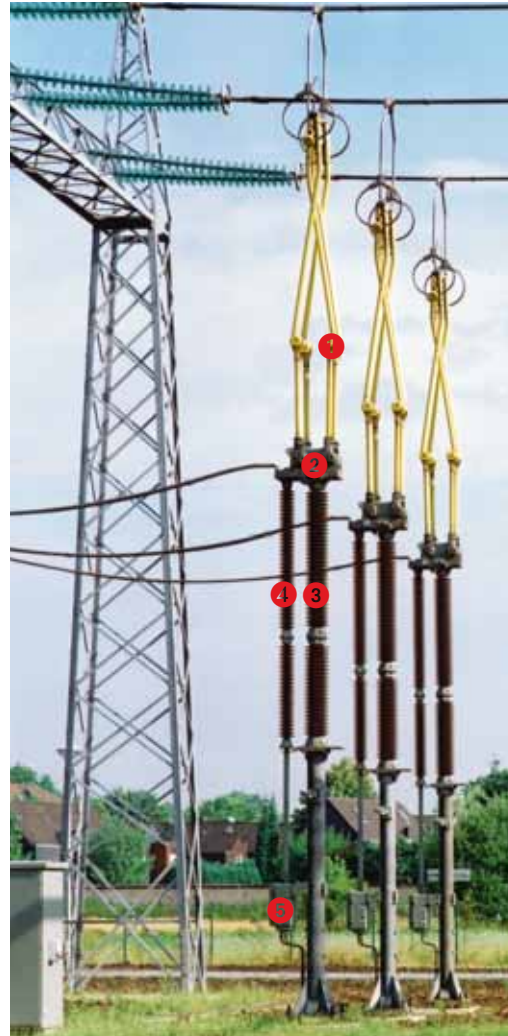
Fig. 4.1-20: Components of the pantograph disconnector
