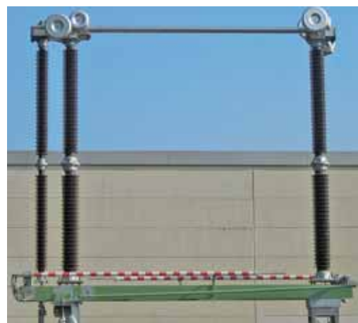
Fig. 4.1-21: Vertical-break disconnector
