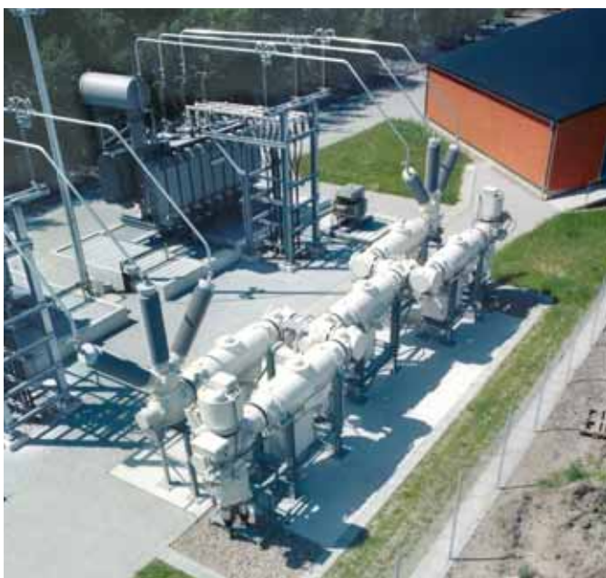
Fig 3.1-27: HIS Substation
