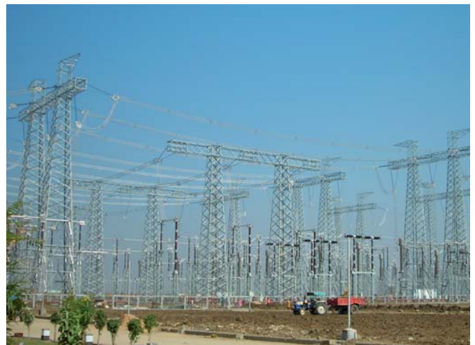
Fig. 3.1-24: One-circuit-breaker-and-a half arrangement, 800 kV, India
