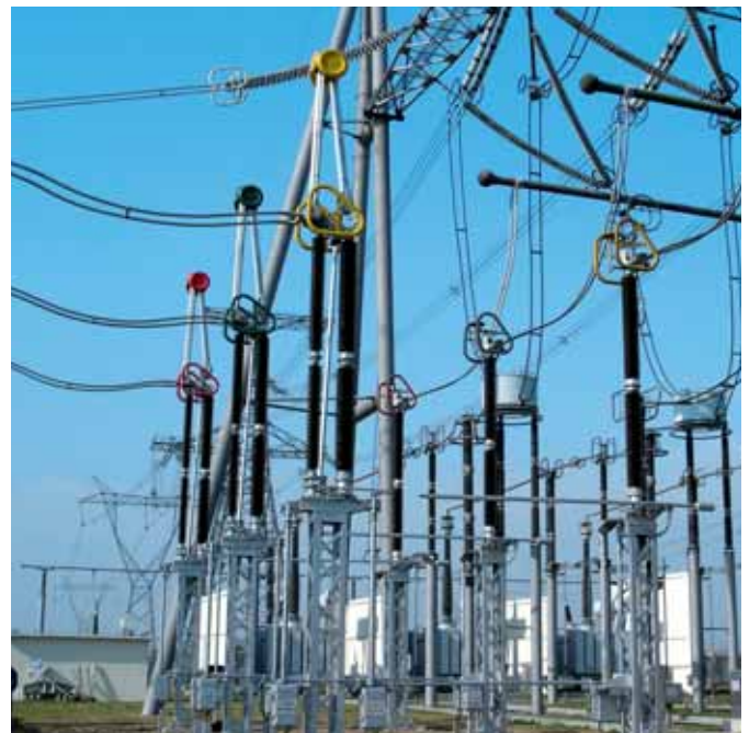
Fig. 4.1-23: Knee-type disconnector
