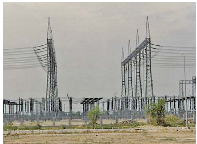
Fig. 3.1-22: One-circuit-breaker-and-a half arrangement, 500 kV, Pakistan
