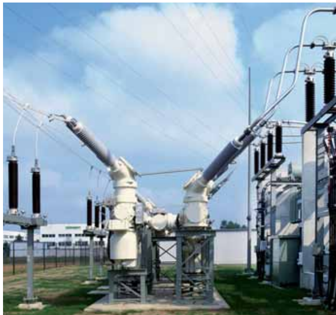
Fig. 3.1-32: H-arrangement with HIS, 123 kV, Germany
