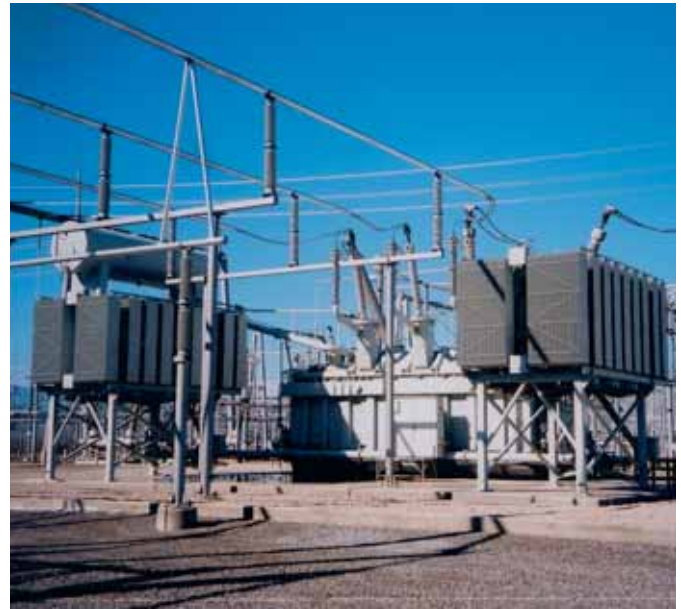
Fig. 5.7-1: Phase-shifting transformer
