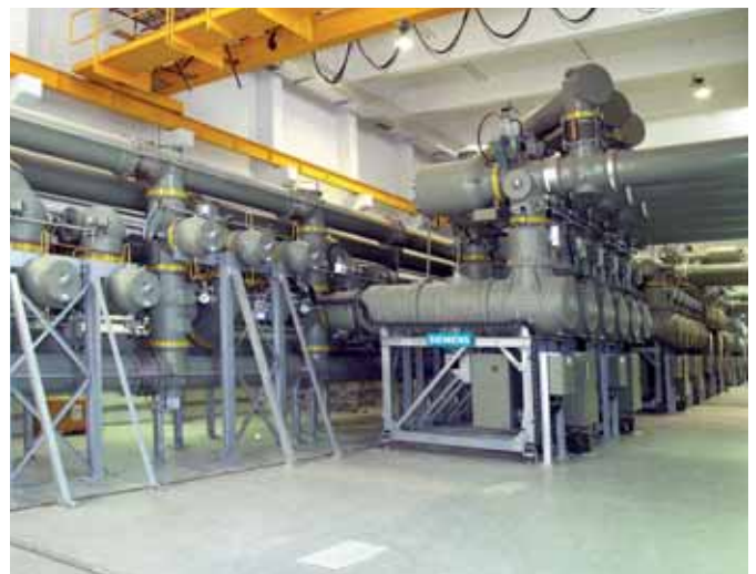
Fig. 3.1-39: 8DQ1 switchgear for a rated voltage of 420 kV
