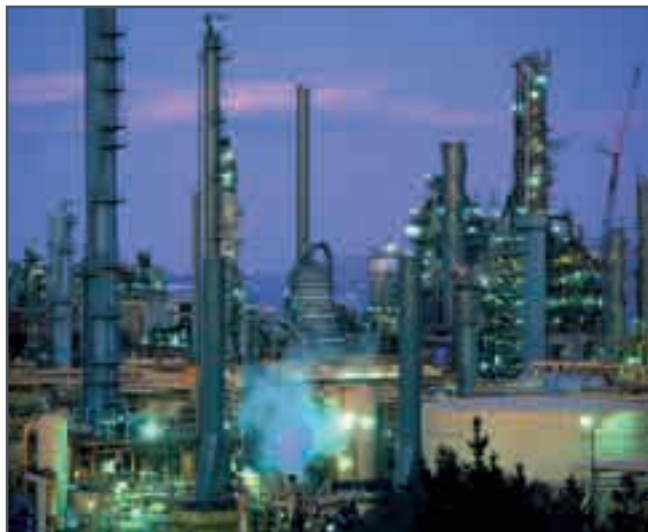
Figure B3.1: Large modern industrial plant
